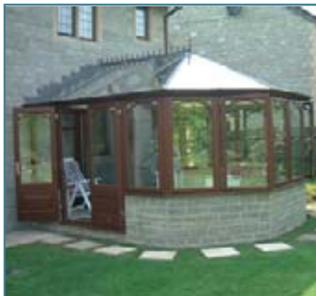
Fig 2 Three bay Victorian design with swept head casements, stained mahogany.
