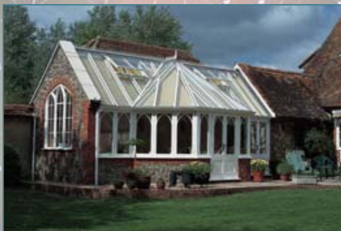
The existing gothic arch window was removed, restored and fitted within a newly built gable.
